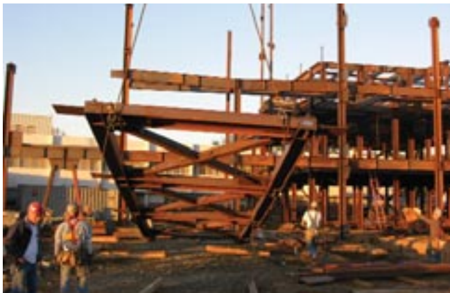
Steel frame going up, February 2005
