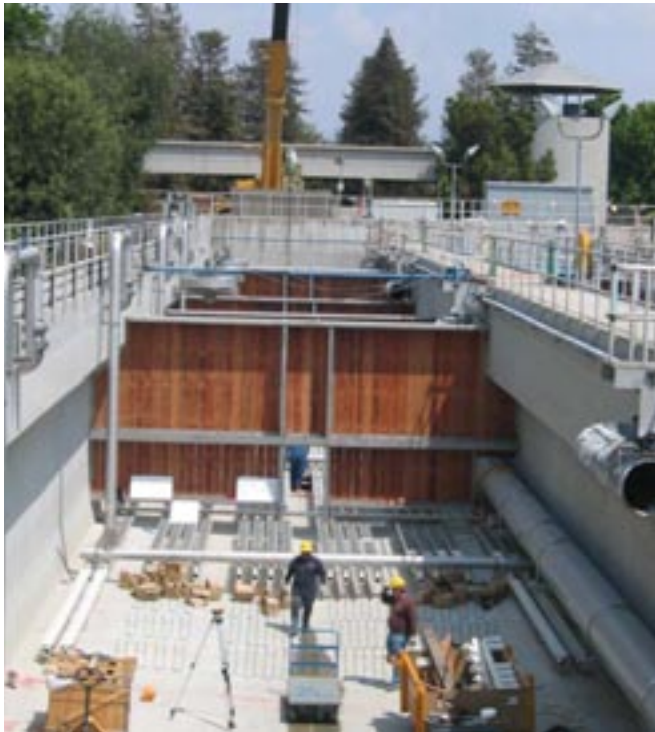
Phase I Aeration Tank #1 Baffle Installation
