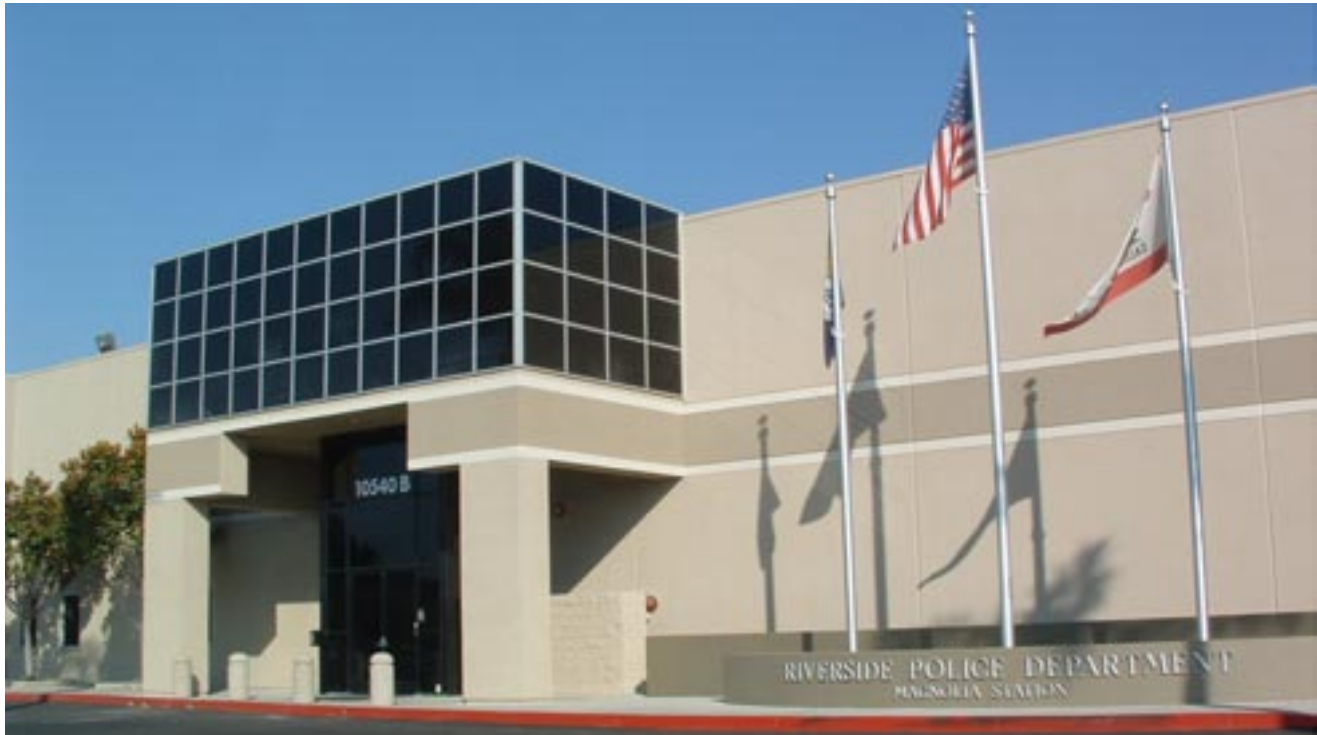
Finished entry monument for the new Magnolia Police Station
