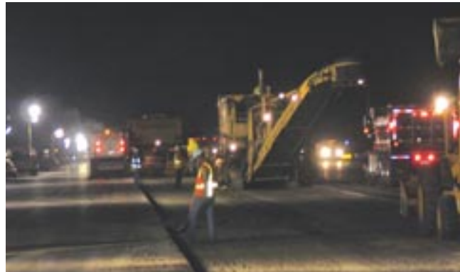
Pavement reconstruction underway for Bob Hope Airport
